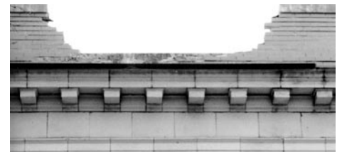
The removed section of the terracotta.
